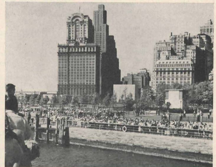
As the Liberty brings a load of visitors back to Manhattan, hundreds are lined up on shore waiting to begin their tour. On weekend afternoons two boats shuttle between Battery Park and Bedloe's Island, one leaving every half hour.
