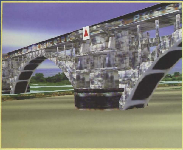
A close-up of the part of the bridge (very dark, touching the water) causing collisions most frequently. Swift currents, bridge span limitations, and the increasing size of the cargo as well as its length will all increase the probability of a collision between the bridge and the pilot's cargo, hence the navigational challenge.
