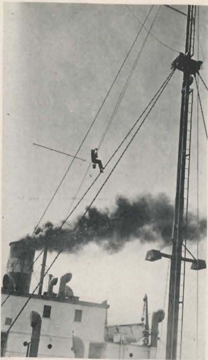
Slushing stays of foremast. An A.B. seaman in a bosun's chair aloft. A tallow and white lead mixture protects the guy stays from rust and corrosion.
