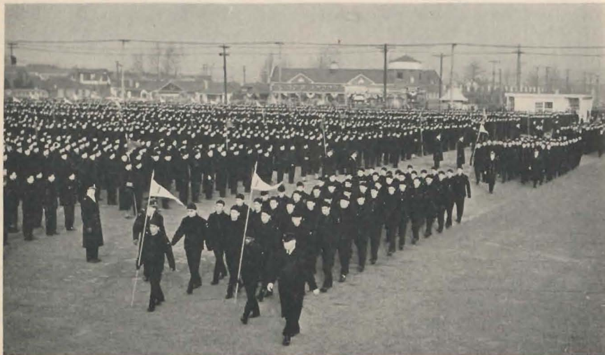
Drilling at World's Largest Maritime Training Station
