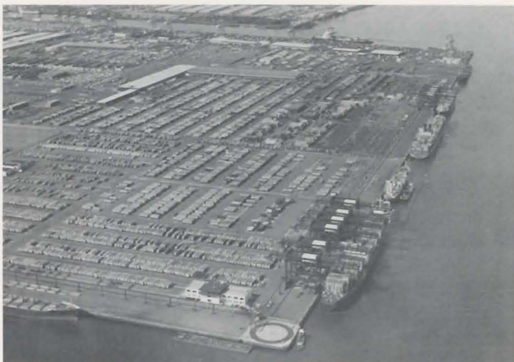
Piers in Port Elizabeth, N.J.
