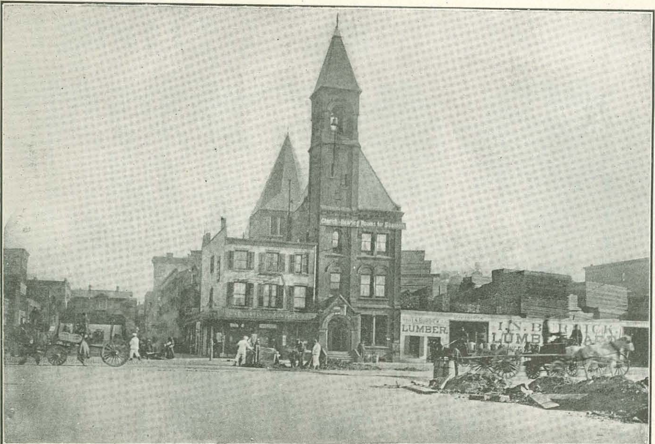
NORTH RIVER STATION Church, Institute and Chaplain's House form an L on West and Houston Streets
