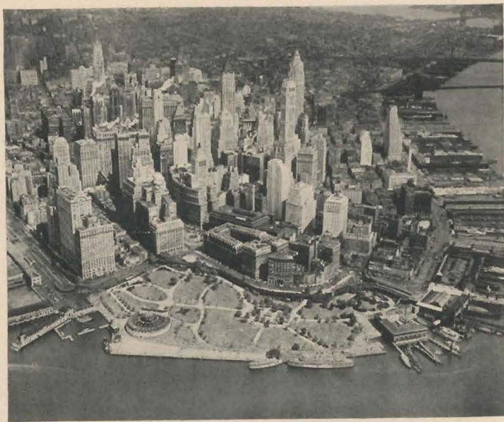
A View of Battery Park, the tip of Manhattan Island, where the North and East Rivers meet. This view was taken in 1942 before demolition began of the Aquarium and of the 6th and 9th Avenue Elevated tracks.
