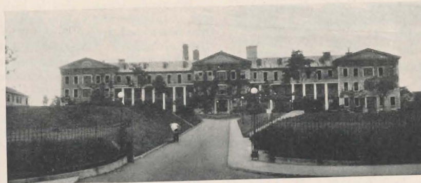
U. S. Marine Hospital at Staten Island, N. Y.
