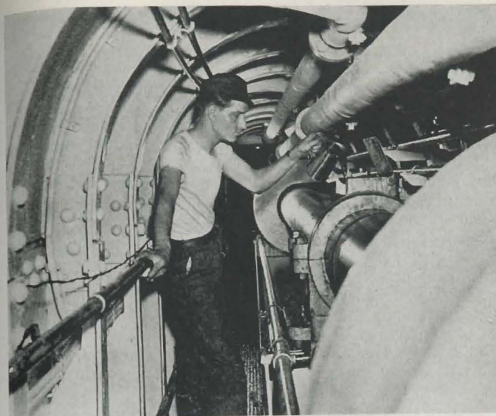
OILER in shaft alley
