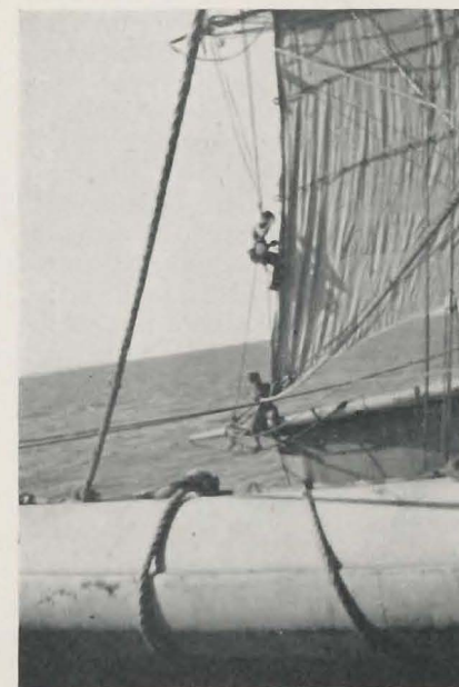
Photo by Elsie Jansen Putting Chafing Gear on Leach of Sail
