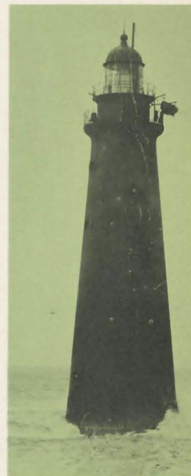
Minot's Ledge light station (Massachusetts) circa 1800's. Completed in 1868.
