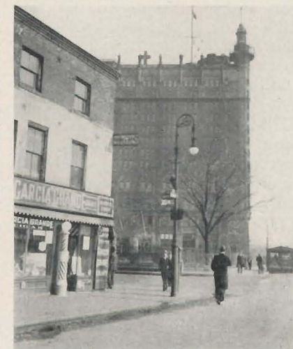
The South Street Approach
