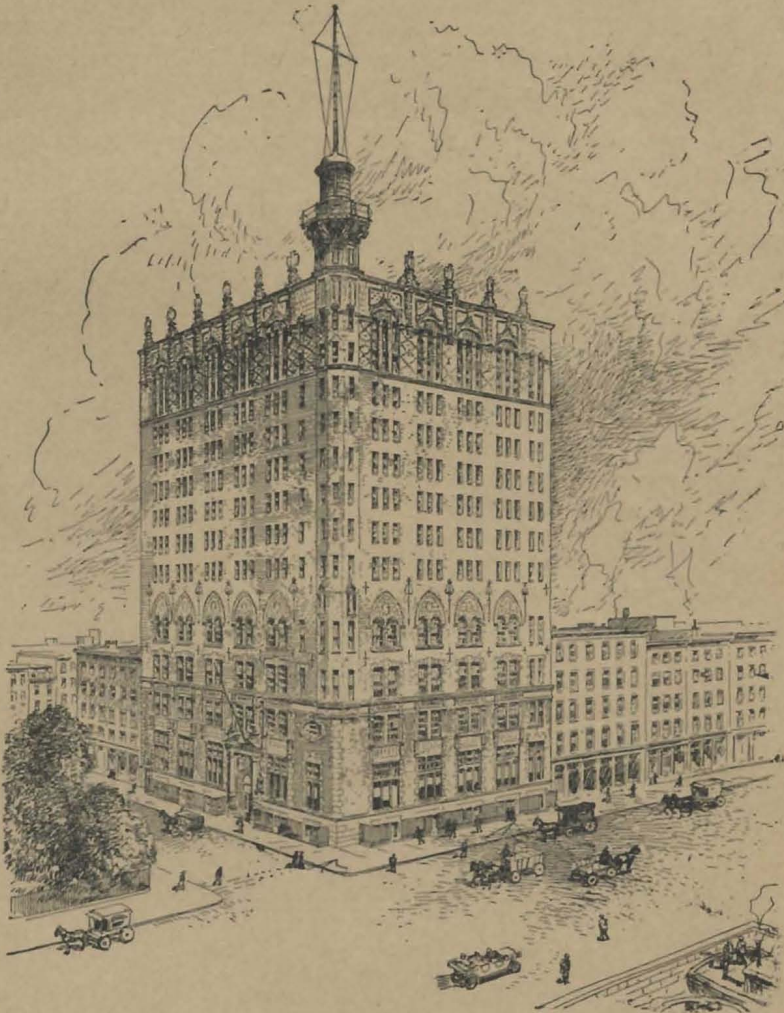
NEW BUILDING Now being erected
