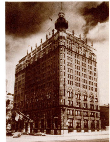
...and atop SCI at 25 South Street
